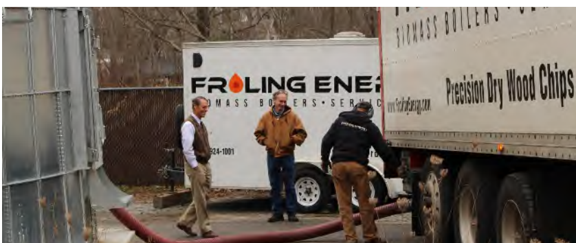
The first blower truck delivery of PDCs into Filtrine's silo.
